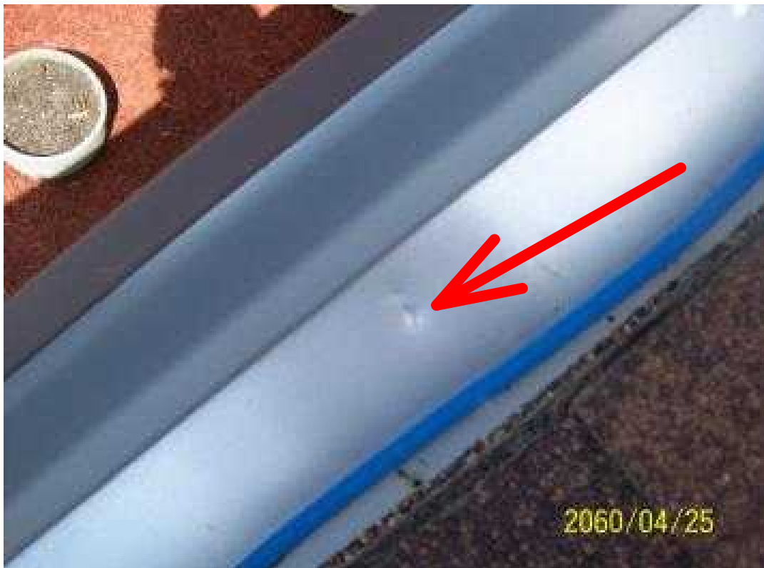
Hits to aluminum eaves troughs
